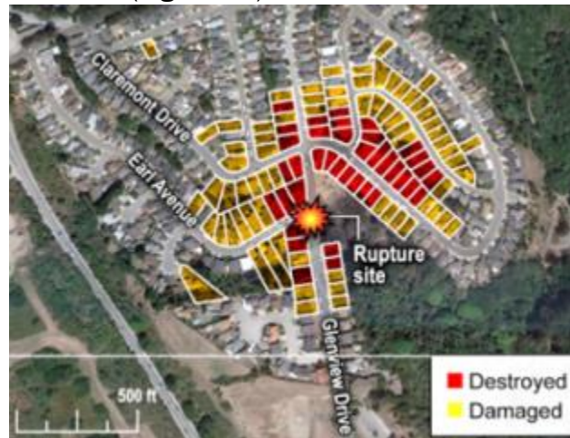
Figure 38: 2010 Natural gas leakage and explosion from underground natural gas pipeline in San Bruno, California. Source: Pipeline and Hazardous Materials Safety Administration.
